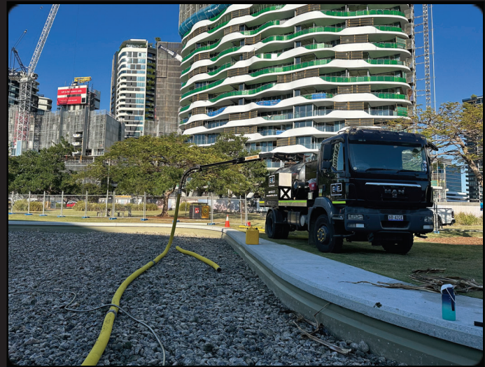
NDD Footing Excavation & Investigations
